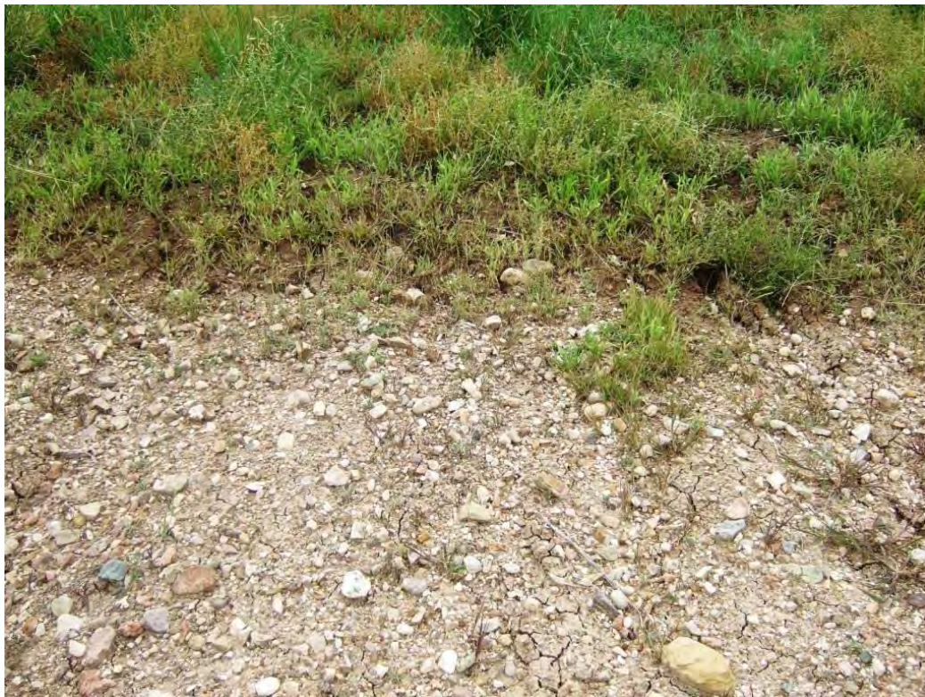
Plate 12: Exposed soils on dam wall in Survey Unit 5
